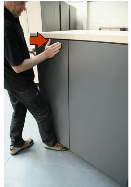
3. Push the top clips into place then go over the whole panel again ensuring contact along all edges. DONE
