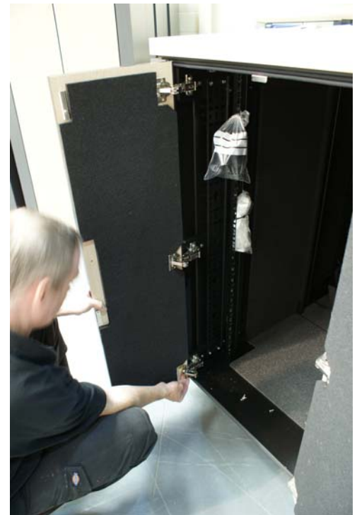
6. Fix the two screws holding each hinge onto the doors, starting from the top and working down. DONE.
