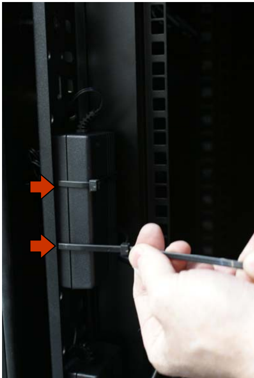
4. Secure the PSU firmly in place with the two large cable-ties.
