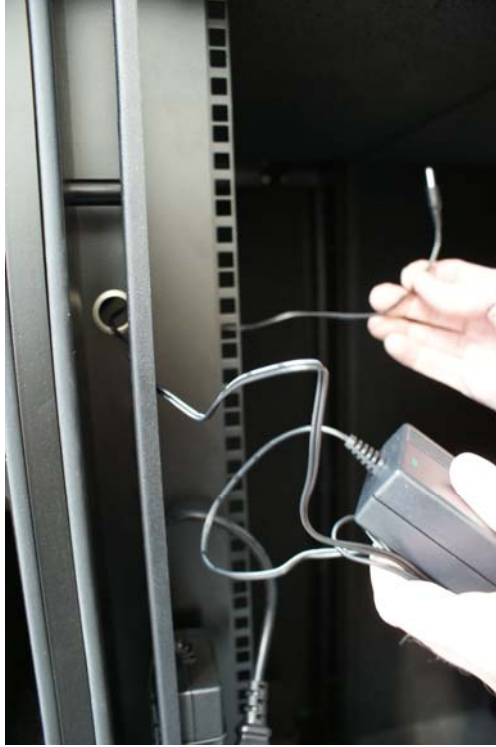
2. Thread the Jack through the cable-tray and into the cabinet through the hole provided.
