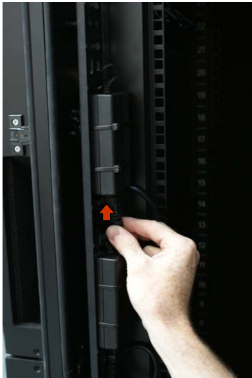
5. Reconnect the power cable to the PSU. DONE.
