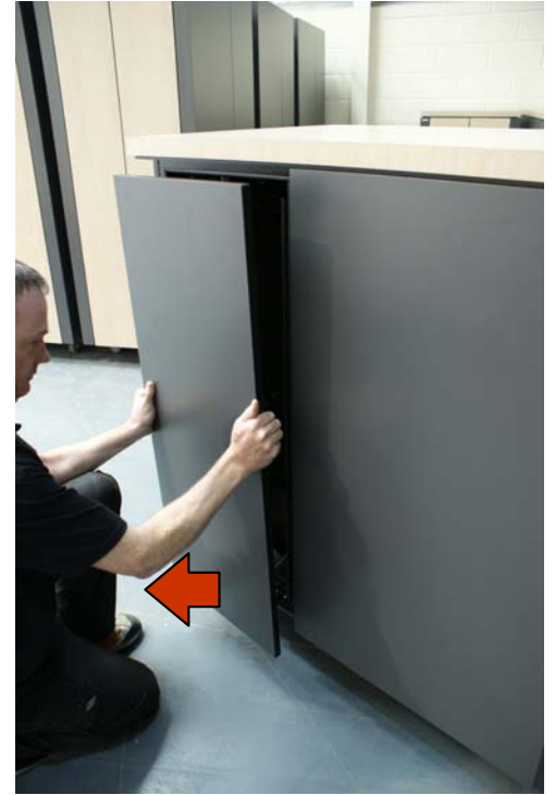
3. Working your hands down the panel, lever the remaining clips free and remove the panel
