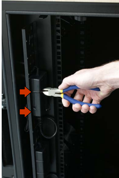
2. Snip the cable-ties holding the PSU in place
