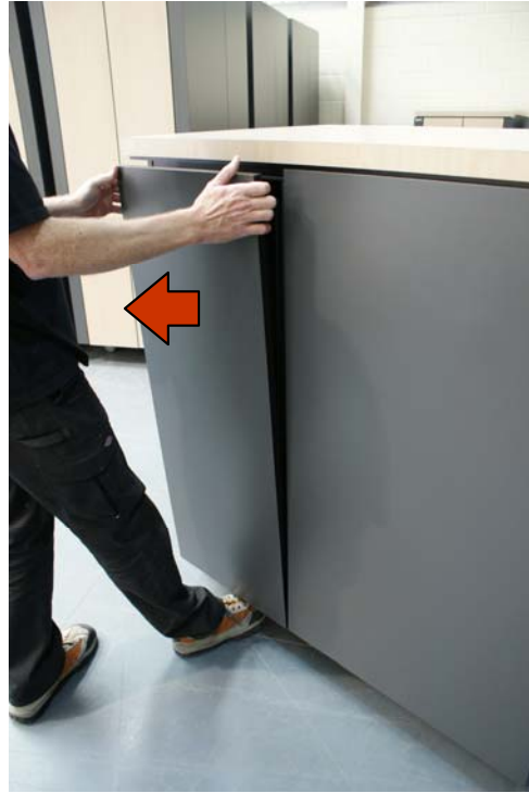
2. Work the top forward corner free
