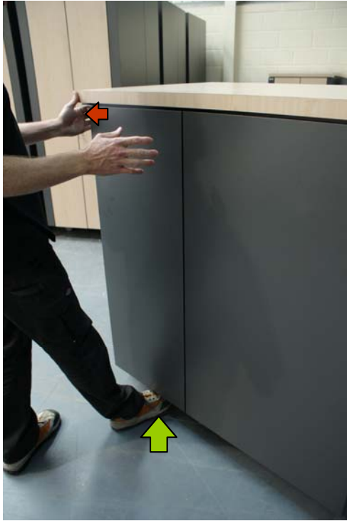
1. Pull the top rear corner of the panel free, supporting the panel underneath with your foot
