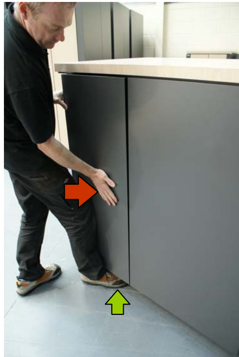
2. Keeping the bottom pushed in, work your way up the panel
